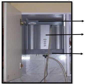
Size of RO with filters need to be considered before constructing cabinet.
