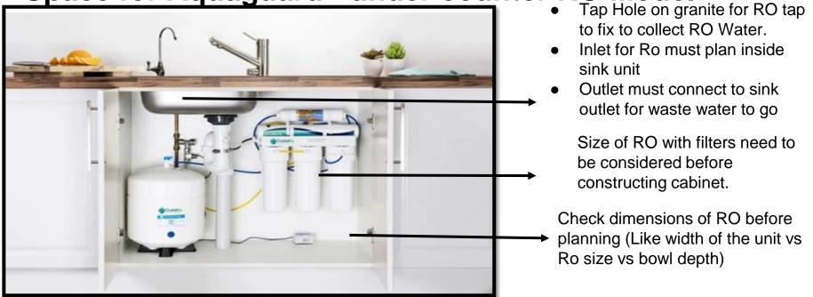
\*Note: Electrical and plumbing inlet and outlet points should be considered near to RO.
